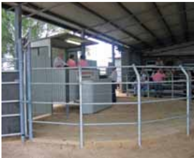
This sale ring is provided with a barrier to enable the handler to step behind when cattle are in the ring.
