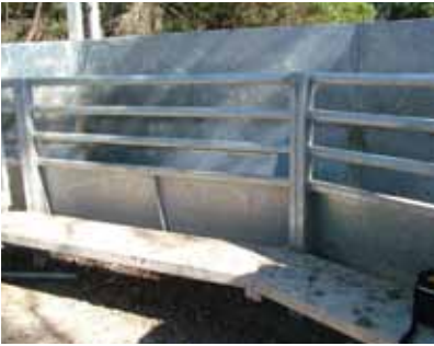
A non-slip concrete catwalk beside the race.
