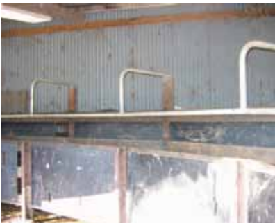
A race top rail supported from above to enable clear access through the rail for injecting.
