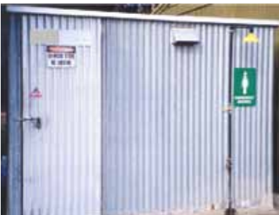
Farmer-constructed lockable chemical store. Includes bunded concrete floor, ventilation and emergency deluge shower.
