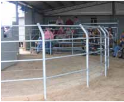
A well constructed sale ring with the top of the fence angled at 45 degrees.
