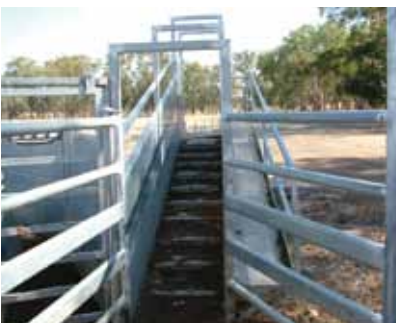
Loading ramp with catwalk attached to the ramp.
